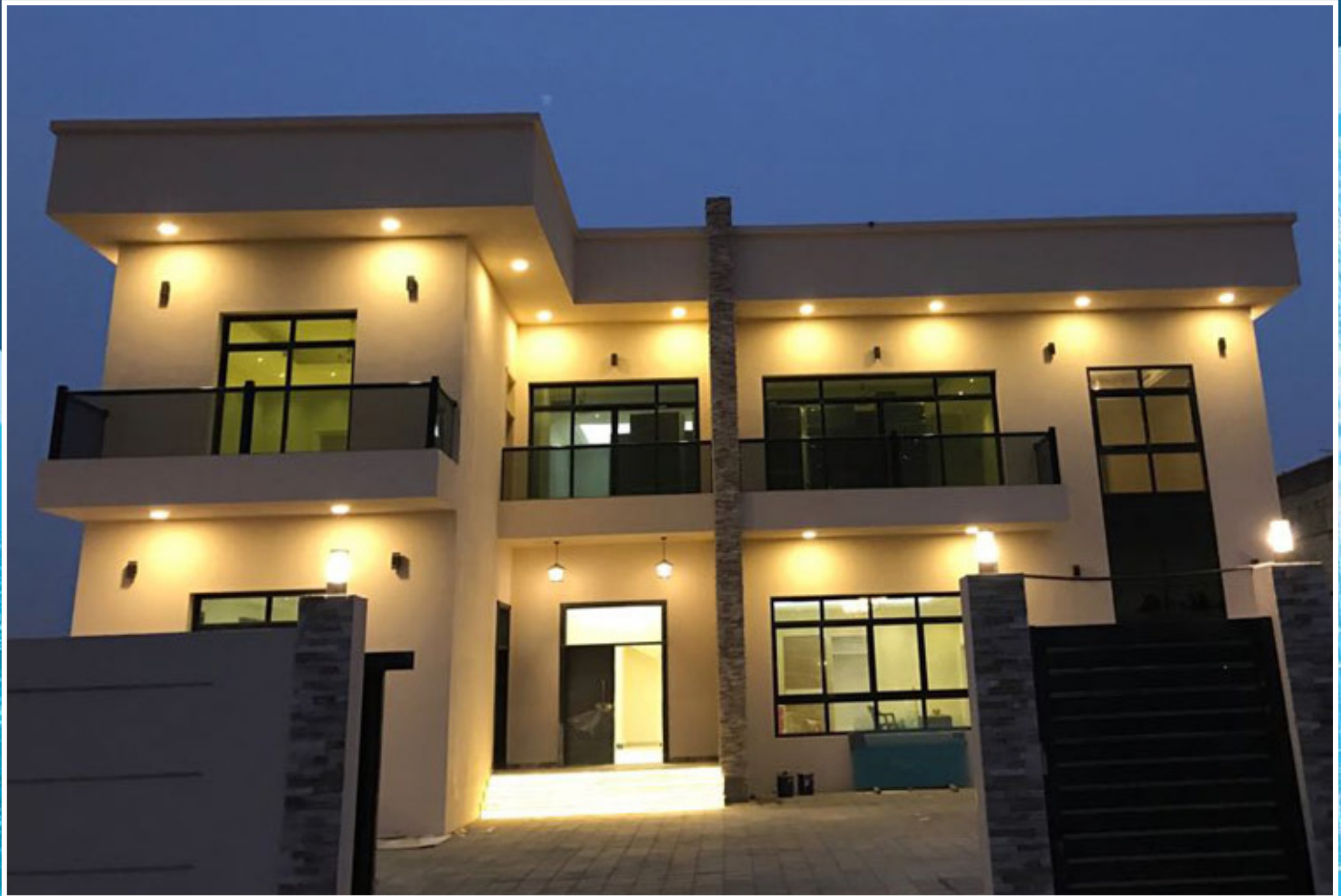
G+1 Villa and Compound Wall at Al Khawaneej Second, Dubai.
