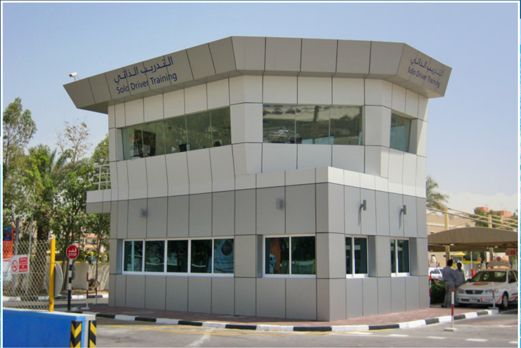
Construction G+1 Building, Solo block and Safety Barrier at Al Qusais and Al Quoze, Dubai.
