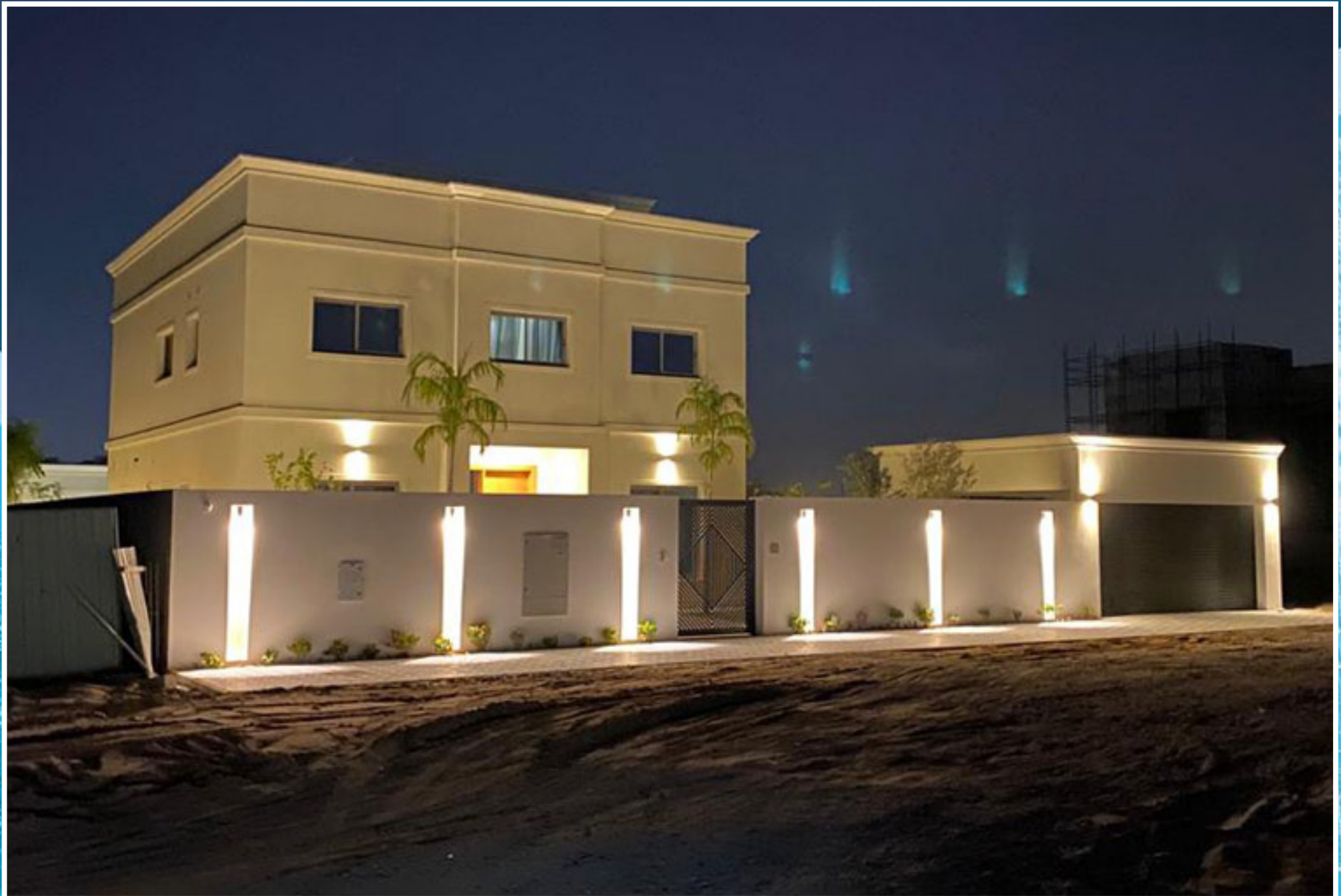
Residential Villa (G+1) at Al Khawaneej Second, Dubai.
