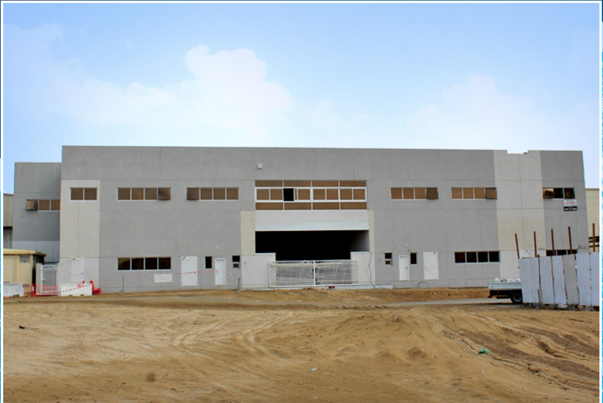
G+M Warehouses (6nos.) at Al Qusais Industrial Fifth, Dubai.
