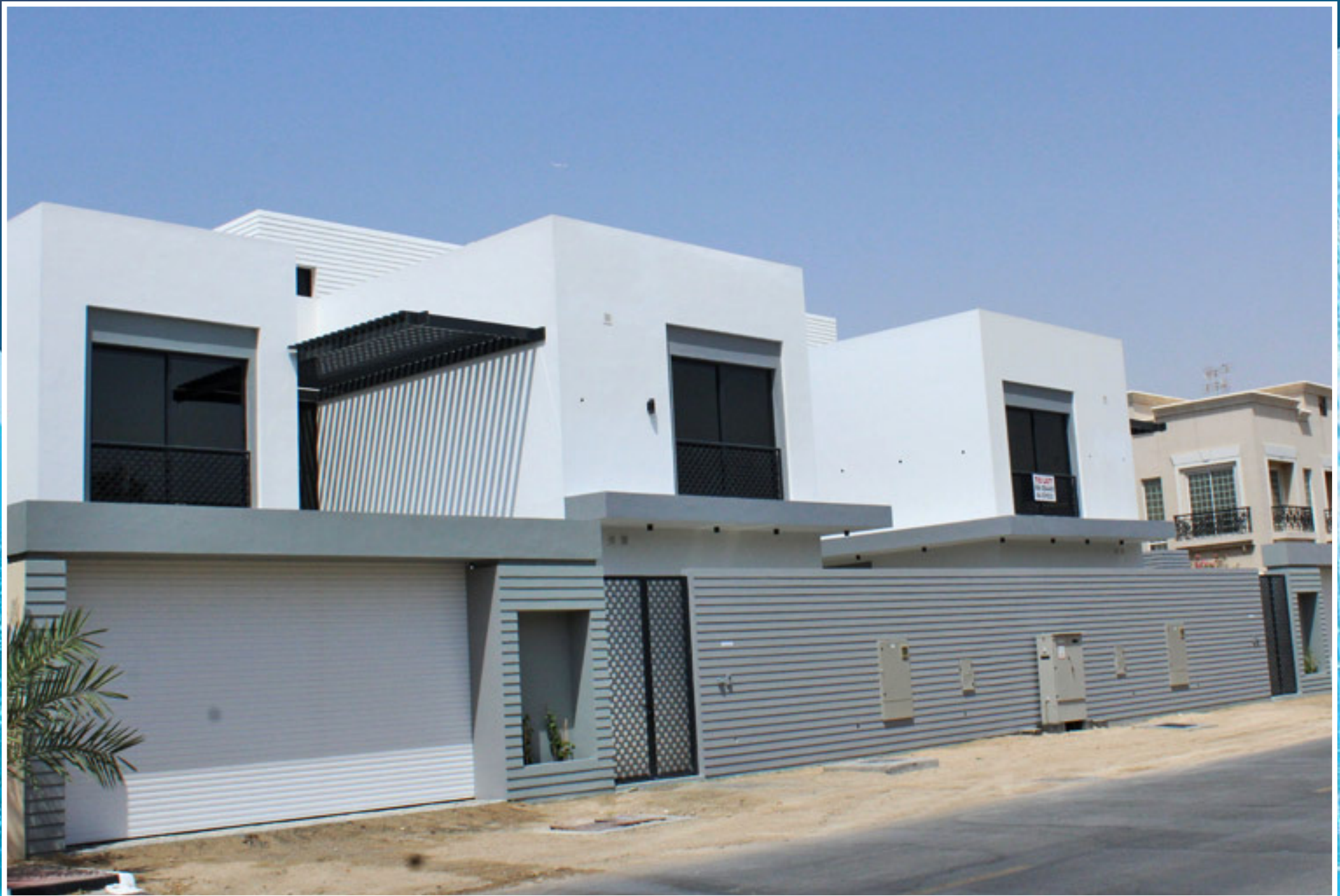
G+1 Twin Villa at Al Manara, Dubai.
