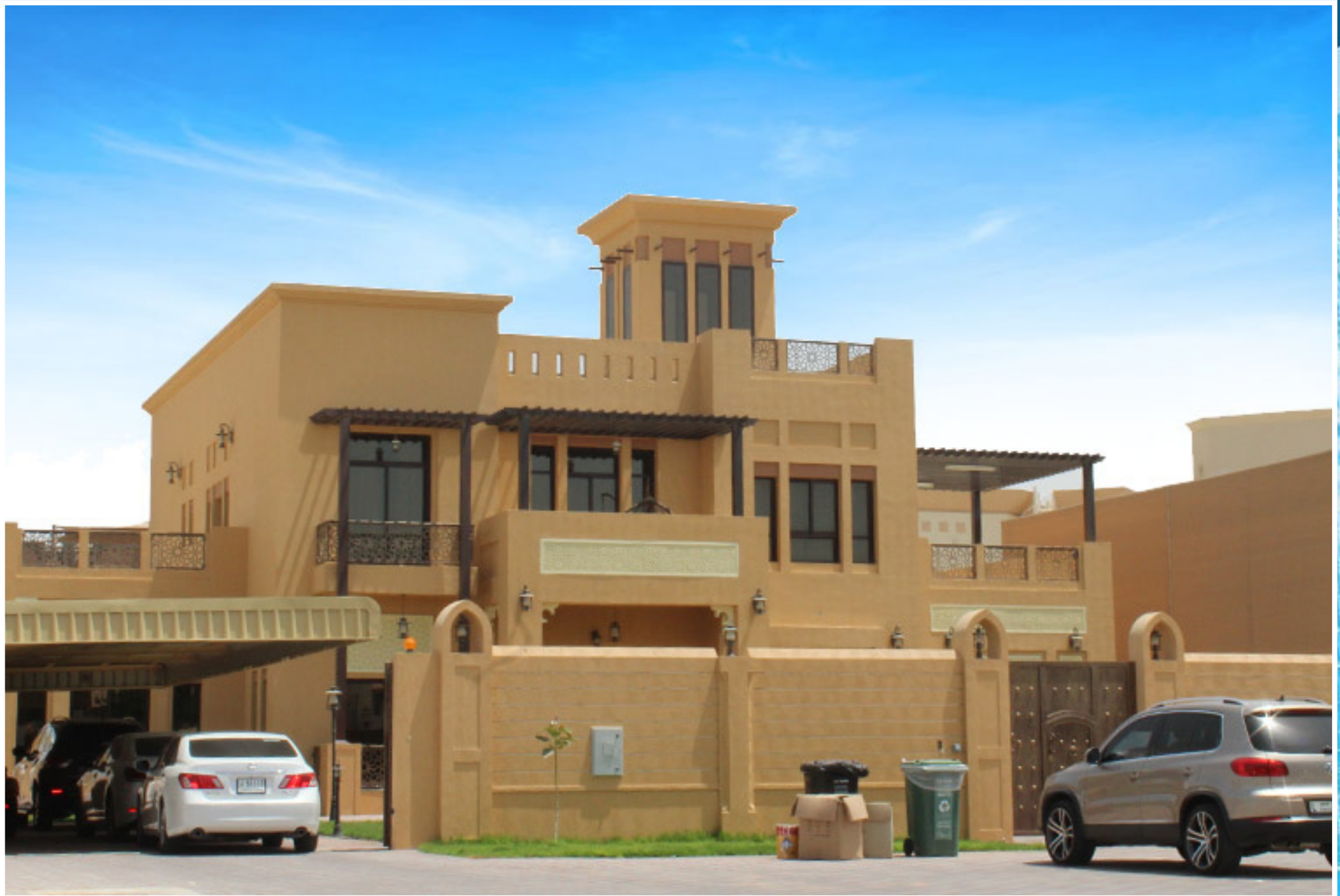
G+1 Villa and Service Block at Umm Suqeim First, Dubai.
